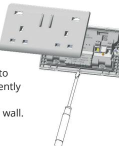
2. Place a suitably sized flat bladed screwdriver into this slot and gently lever the plate away from the wall.
